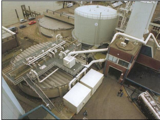
Then it was seeded with waste activated sludge. The flow was gradually increased in stepwise increments. At seven weeks the reactor was at full flow and load. (See **Figure 7. "INCREASE IN LOAD OVER TIME"**)
