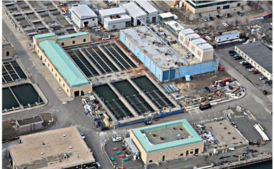
At the Wards Island biosolids processing complex, centrate from the centrifuge building (upper left) is sent to the SHARON building (light-blue-walled building on right). There, ammonia is converted to nitrogen gas after caustic soda and methanol are added.
